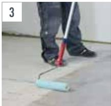
3 Apply an even coat of UZIN PE 360 PLUS primer using a short-pile lambs wool roller or the UZIN nylon fibre roller. Allow to dry for approx. 30–60 minutes.
