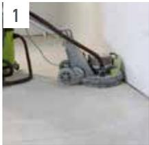
1 Grind the area with a WOLFF grinding machine to remove poorly adhering residues and dirt.
