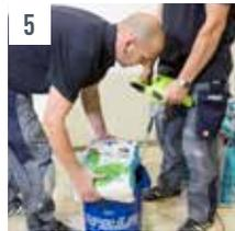
5 The amount of dust generated when opening and mixing UZIN NC 170 LevelStar can be reduced by using a UZIN Ripper and a powerful WOLFF Mixing Drill such as the Power X 1300.
