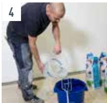
4 Mix UZIN NC 170 LevelStar levelling compound with clear, cold water.
